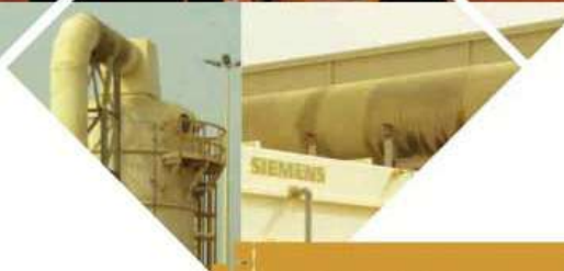
GRP TANKS ERECTION
